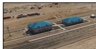
Railroad station Length – 6,8 km. Capacity – 2,3 млн. t/y.
