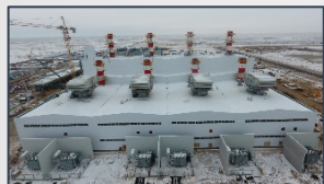
Power plant Output – 310 MW
