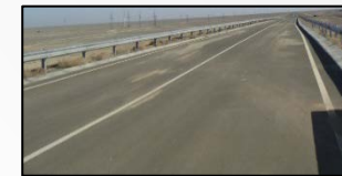
Access road Length - 5,3 km.
